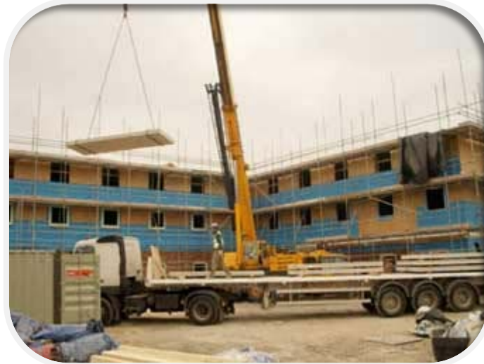
Bison beams being installed onto Hemsec SIPs structure
