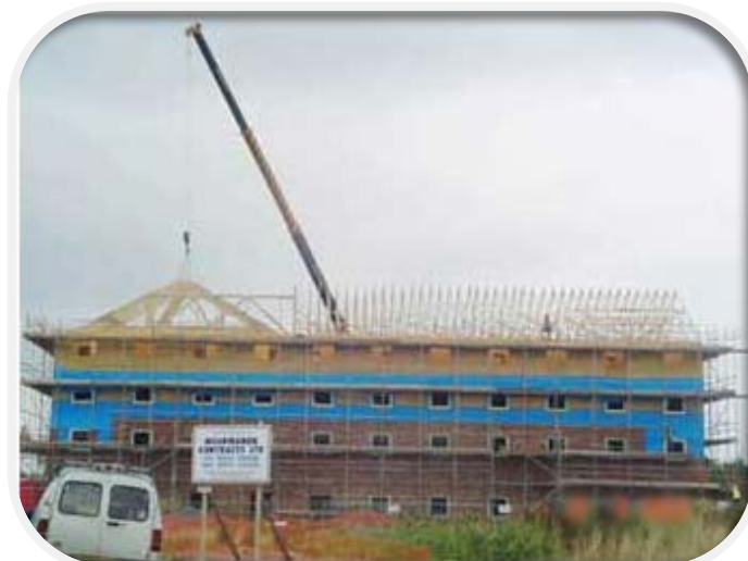
Trussed roof being installed directly onto the Hemsec SIPs structure.
