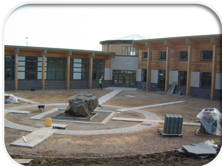
View of the front entrance near to completion.
